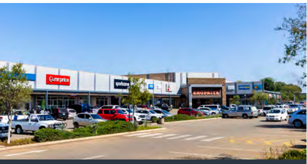
Komatipoort Shoprite Centre Expansion Komatipoort, Mpumalanga | 1 200 m 2 | Opening 1 Nov 2026
