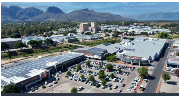
Rembrandt Mall Redevelopment Paarl, Western Cape | 19 387 m 2 | Opening Nov 2026
